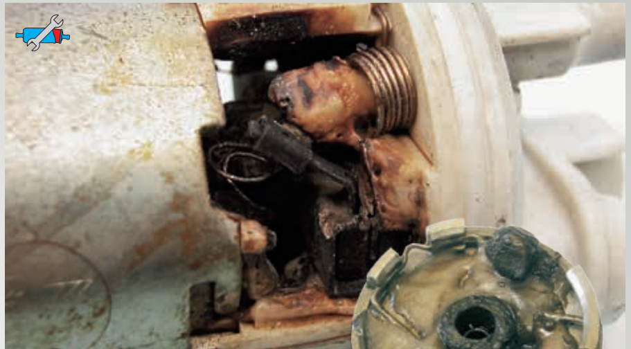
Fig. 20: Friction welding caused by dry running
